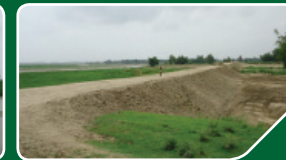
Spur and Soil Embankment (Source: Paudel R.)
