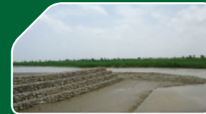
Spur and Soil Embankment (Source: Paudel R.)
