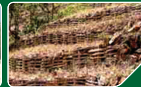
Bamboo plantation in river bed and Bamboo Wattle (Source: IDS-Nepal)
