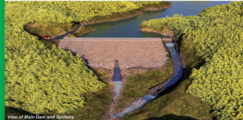
View of Main Dam and Spillway
