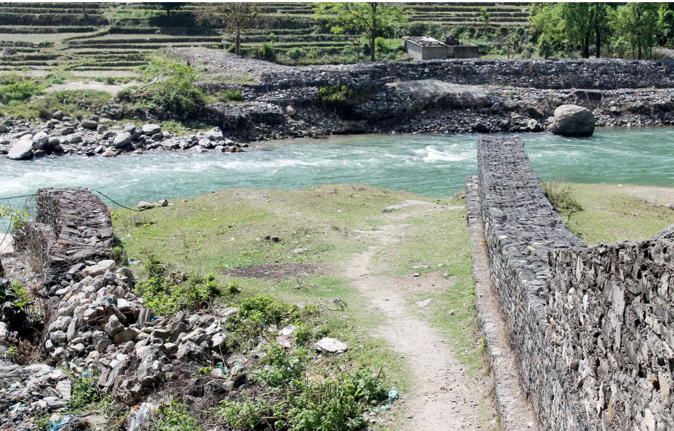
Image 15: Gabion boxes near the river
