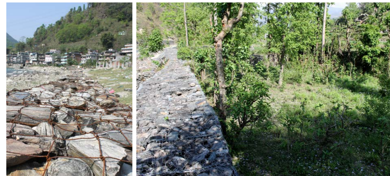
Image 16: Gabion boxes next to the river and on the hillside
